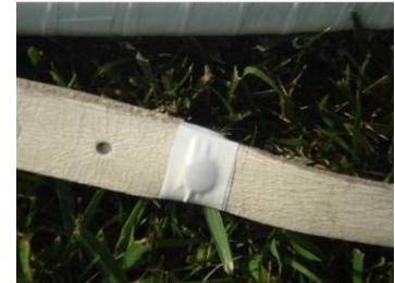
Reattach the bolt and strap. Then cover over the strap screws with a strip of electrical tape in a color that matches the strap.
